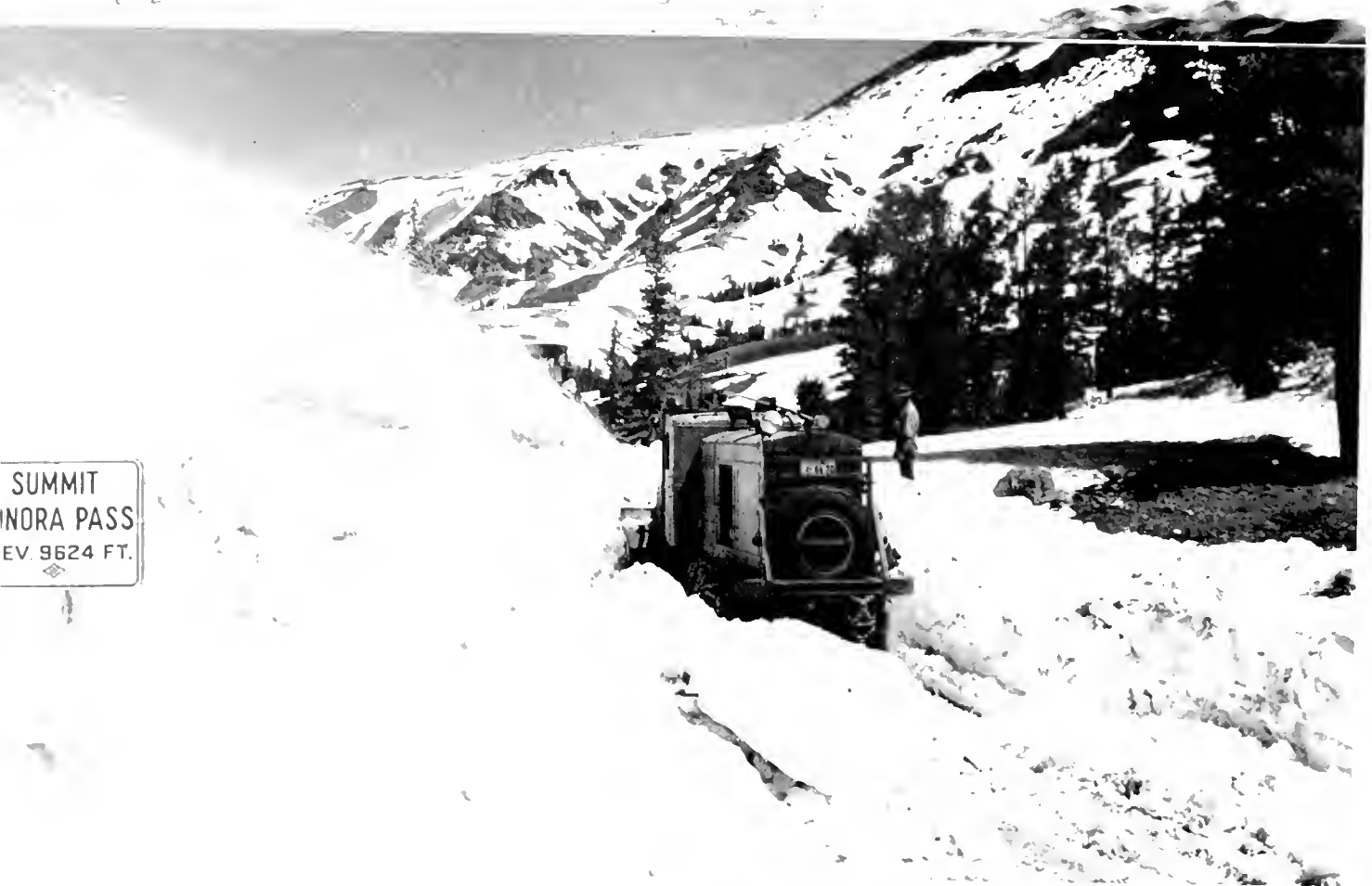
Snow was packed so hard on Sonora Pass Highway that it had to be dynamited before plows could work. Upper—Blowing Pack. Lower—Plow makes headway
